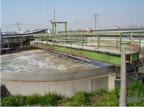
A 600-ton round tank is used for aeration. Liquid portion of hog excreta (wastewater) registers BOD approximately 4,500 ppm.
