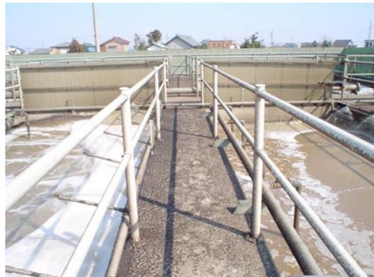
After the first aeration tank, wastewater goes through 6 full-time aeration tanks, 2 intermittent aeration tanks, and a full-time aeration tank to facilitate flock formation.
