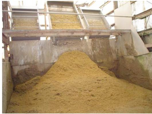
Wastewater goes through two rows of screens on the ground to separate out large solids and fine mesh screens (right picture).
