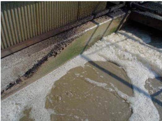
A part of sludge (above picture) is returned to the first aeration tank (see step 4) and to the pits under wooden lattice floor of hog houses.
