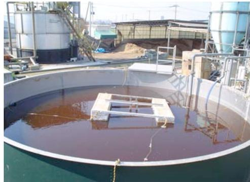
A part of supernatant liquid of sedimentation tank (left picture) is returned to the first aeration tank (see step 4), and other part is forwarded to 100-ton storage tank (right picture) where activated EM is added and returned back to water pools in hog houses.
