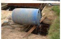
Diluted Extended EM( 1:1000) is dropped into the waste water before the waster entry to the pond.
