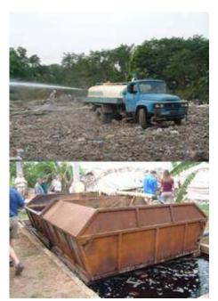
Appling Ex EM for waste treatment : EM : Water=1:100 Spraying dilution of extend EM.
